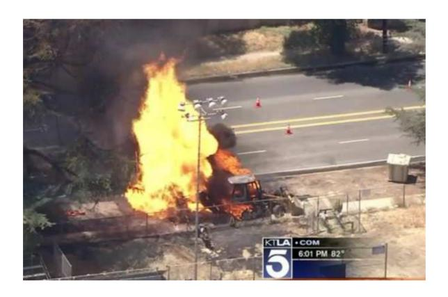
A Los Angeles Department of Water and Power crew was working in the area, operating a backhoe, when the equipment struck a 4-inch plastic gas line.
