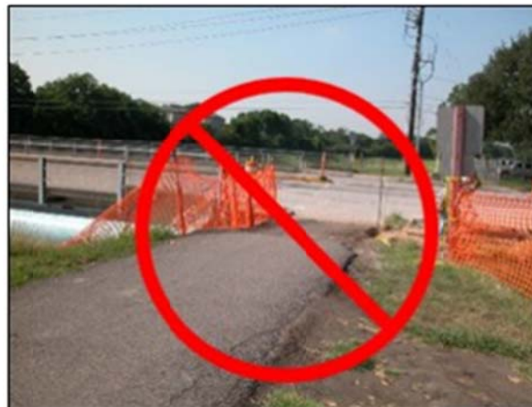
Figure 2 Mesh fencing is not sufficient to protect a pedestrian from falling into a trench or hole
