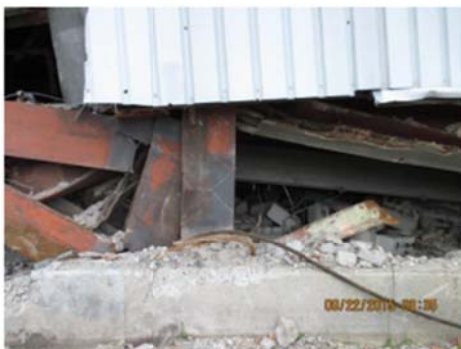
Partial north view FIGURE 15
