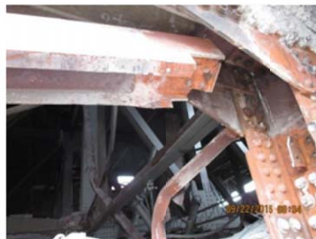
Partial north view FIGURE 16
