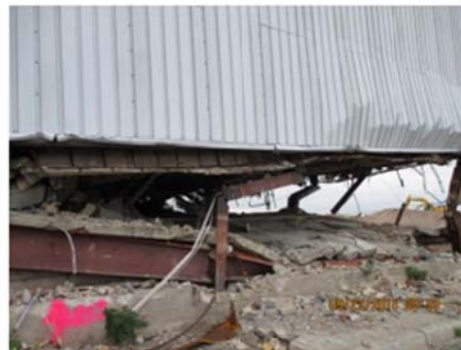
Partial north view from column line A14 FIGURE 14
